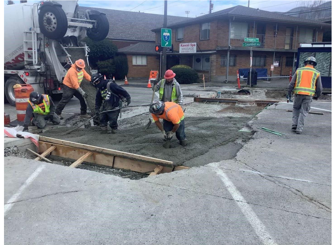
Repaving on 15 th Ave S.
