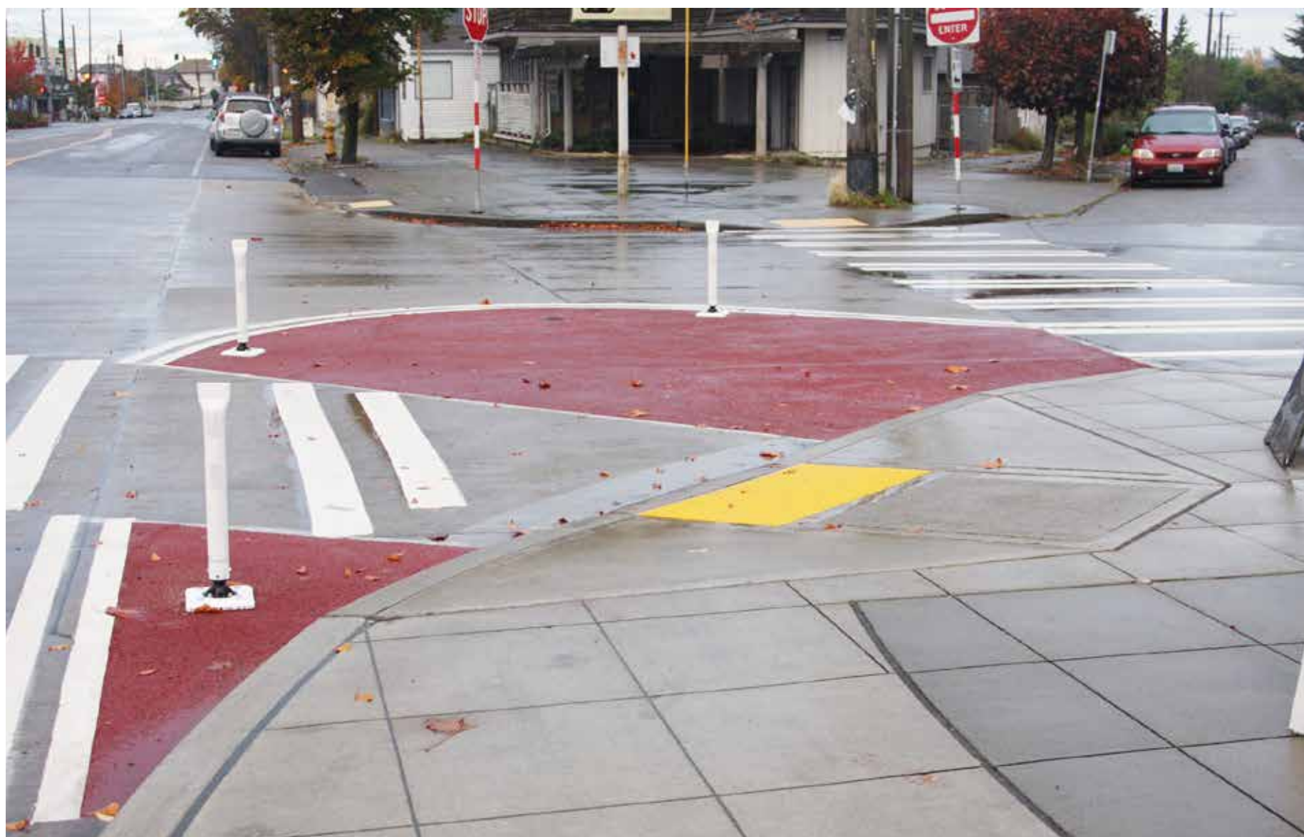
Painted Curb Bulbs (Beacon Ave S/Lander St)
