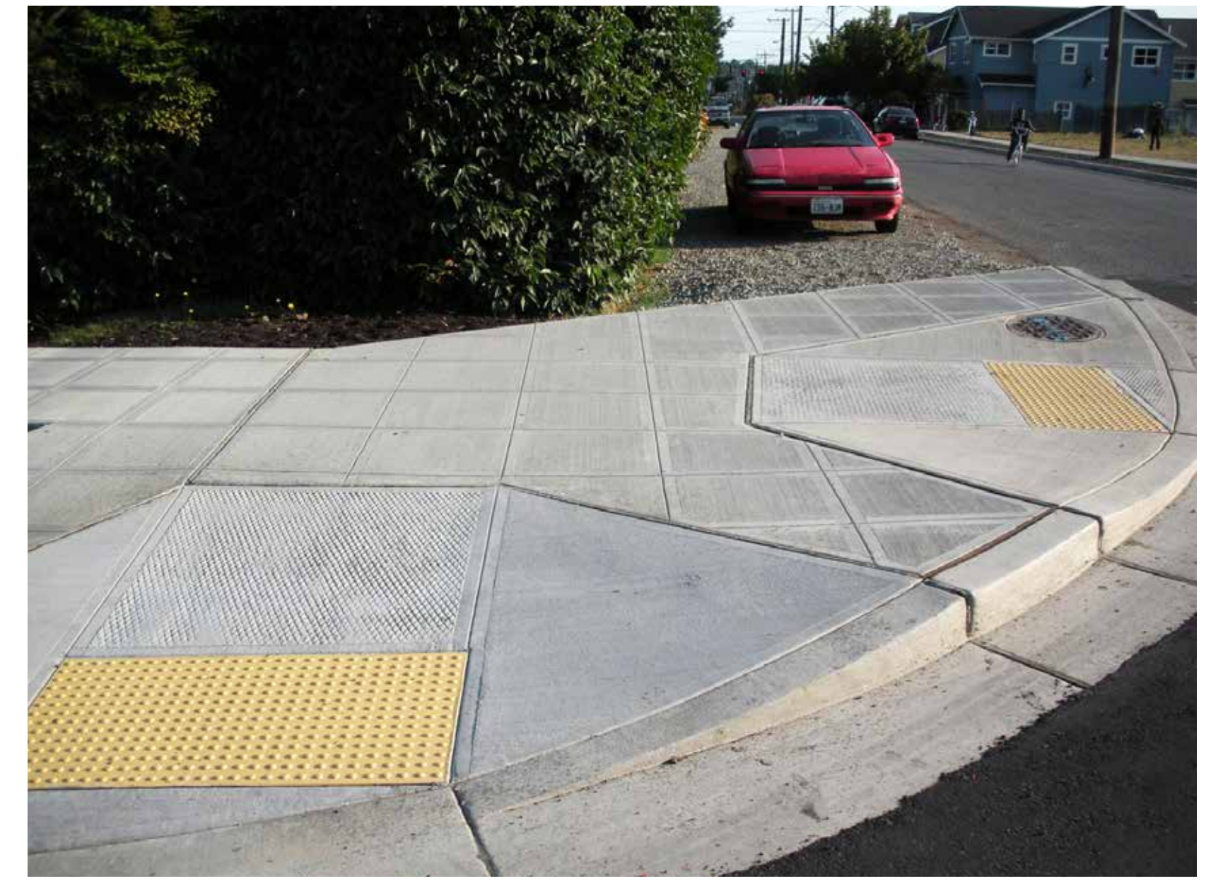
Upgraded curb ramps and sidewalks for people walking and improved ADA accessibility
