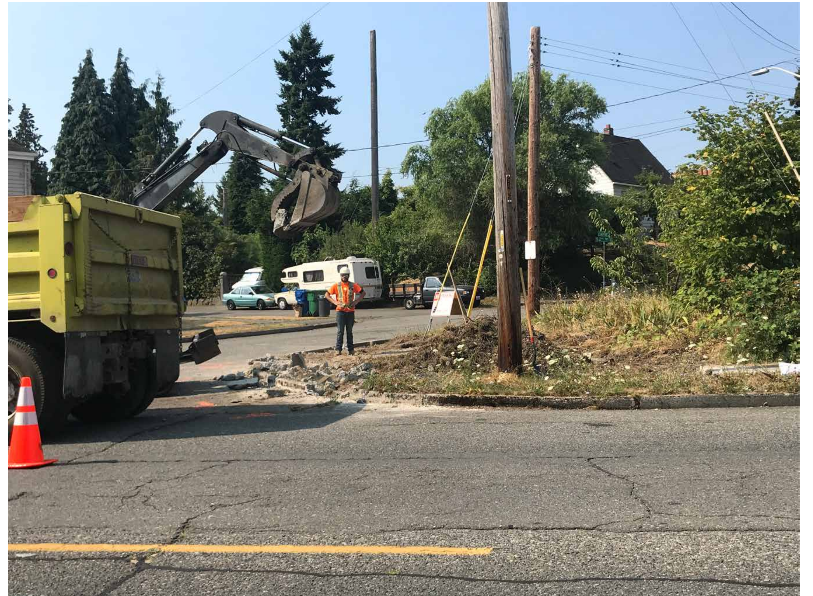
Curb demolition in process.
