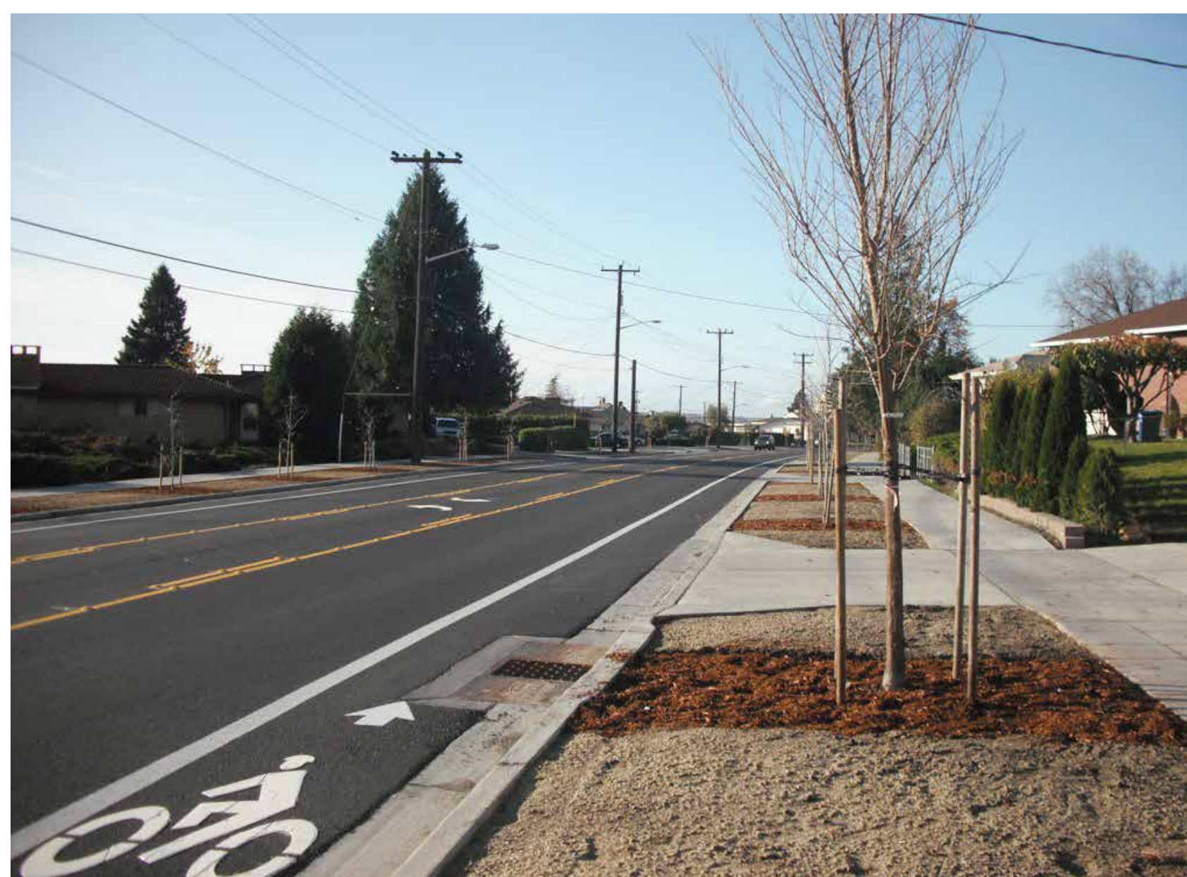
Upgraded stormwater system to filter sediments and pollutants
