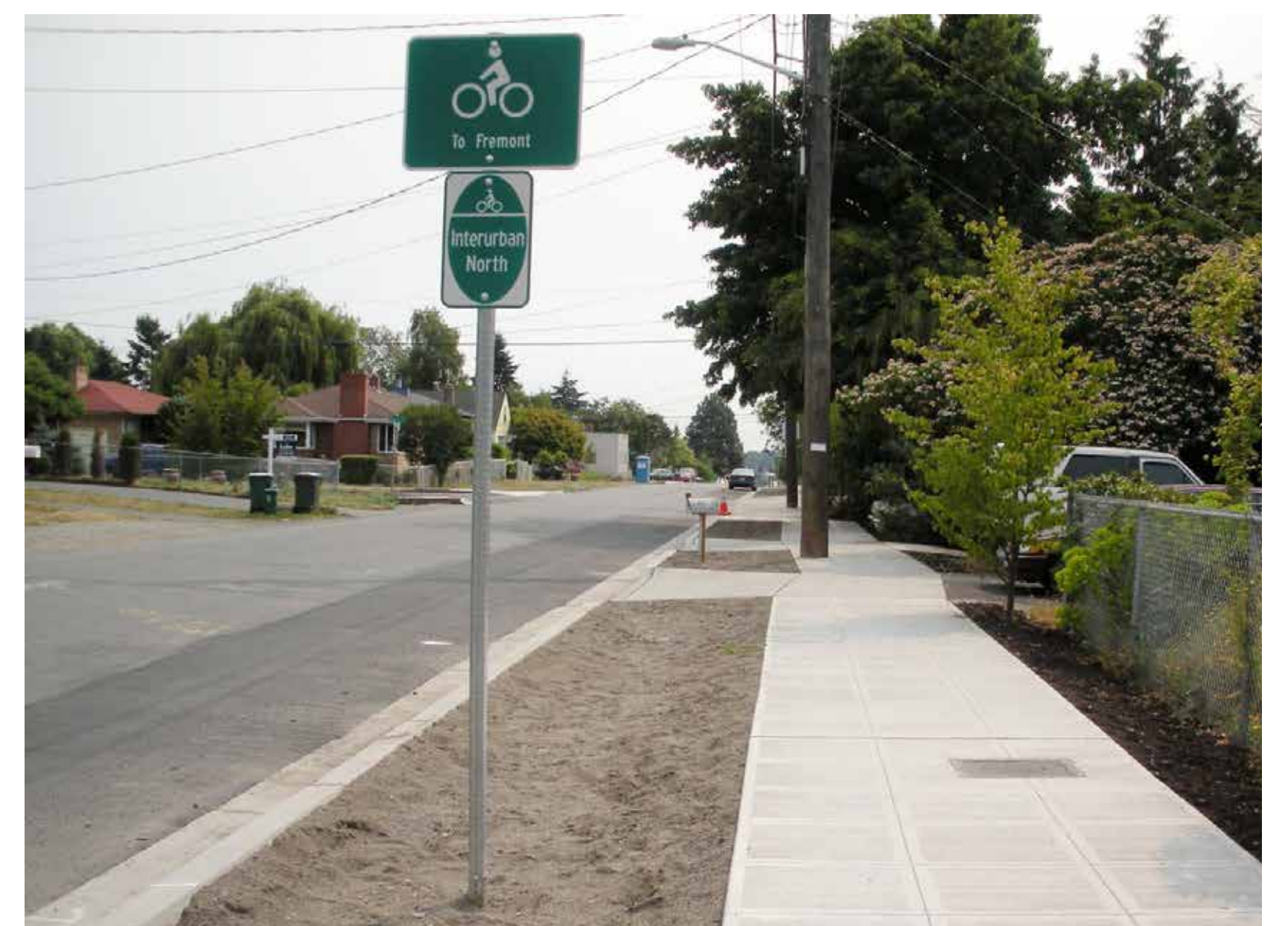
Upgraded sidewalks for people walking
