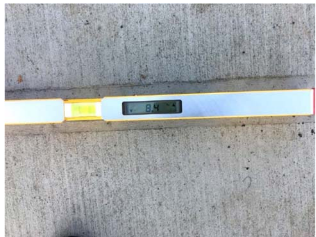
Ramp Running Slope Photo (Example: CR-46thAveS-SHudsonSt_NW-2)
