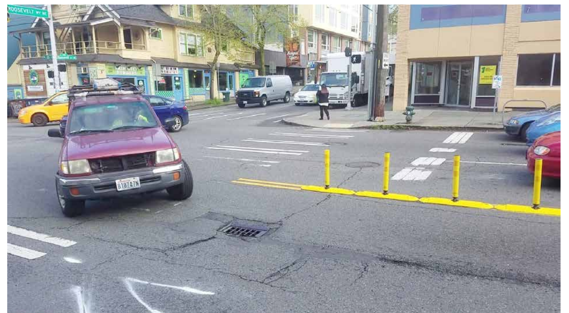
Centerline median with posts at NE 65th St and Roosevelt Way NE
