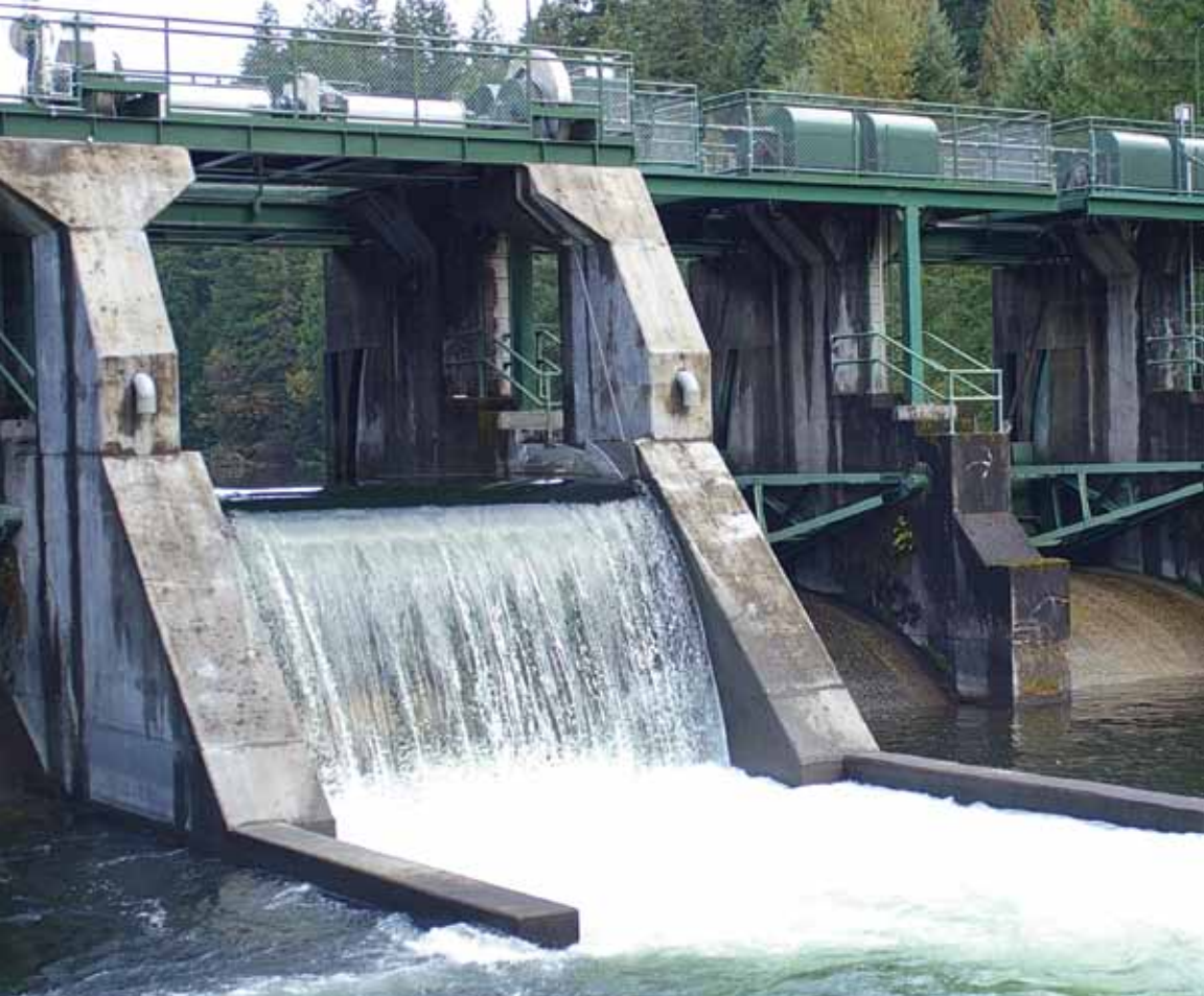
Landsburg Diversion Dam, first built in 1901.
